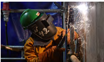
⌘ Welder working in the tunnel reclaim of the Quellaveco concentrator plant.
