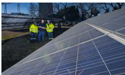
⌘ Our Greenside colliery in South Africa has installed a 90-kilowatt, grid-tied solar farm, which produces enough energy to power all the mine's offices.
